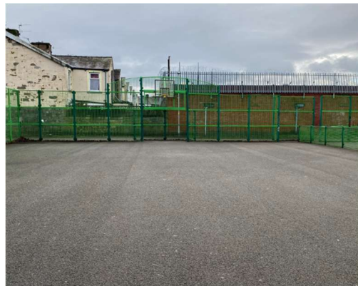
Faded line markings
