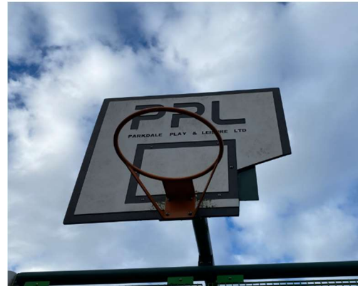
Damaged basketball backboard
