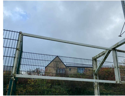
Missing fence panel
