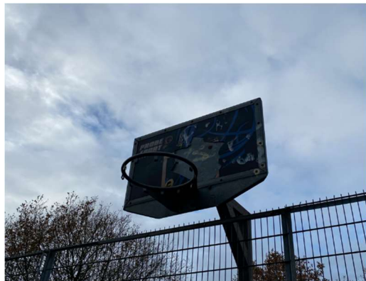
Damaged basketball backboards
