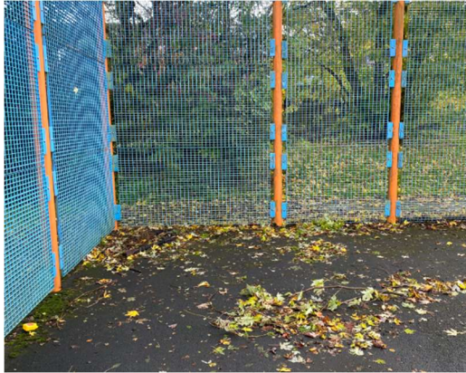
Moss at the corner of the court
