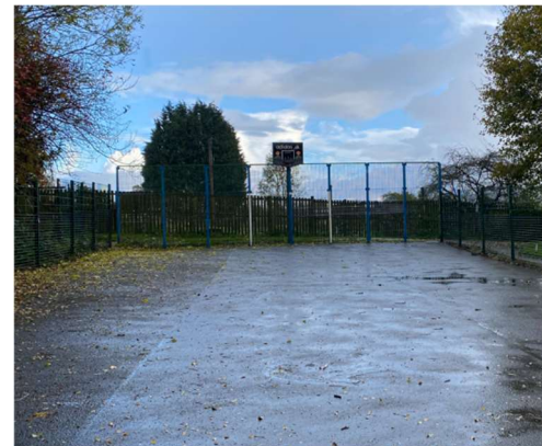
Faded line markings
