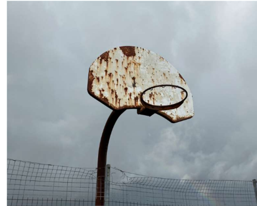
Rusted basketball backboards
