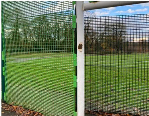
Rust on goal posts
